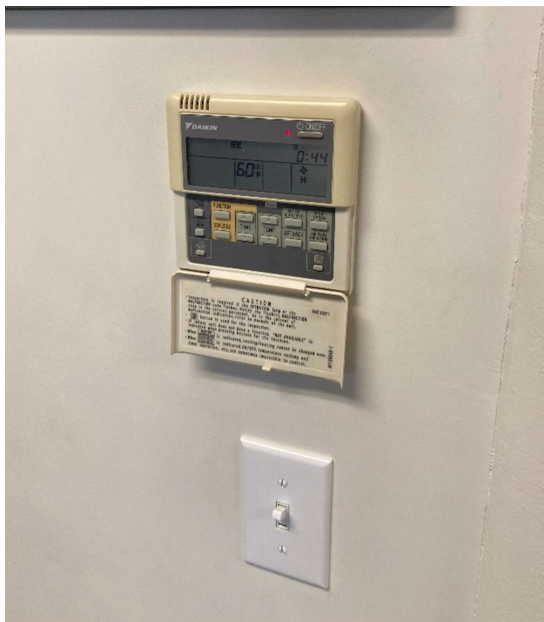
Picture 12: Thermostat for Daikin unit
