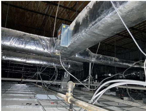
Pictures 6 & 7: Warren electric resistance duct reheat coils located above the drop ceiling.
