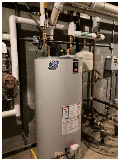
Picture 13: Direct vent propane-fired water heater.
