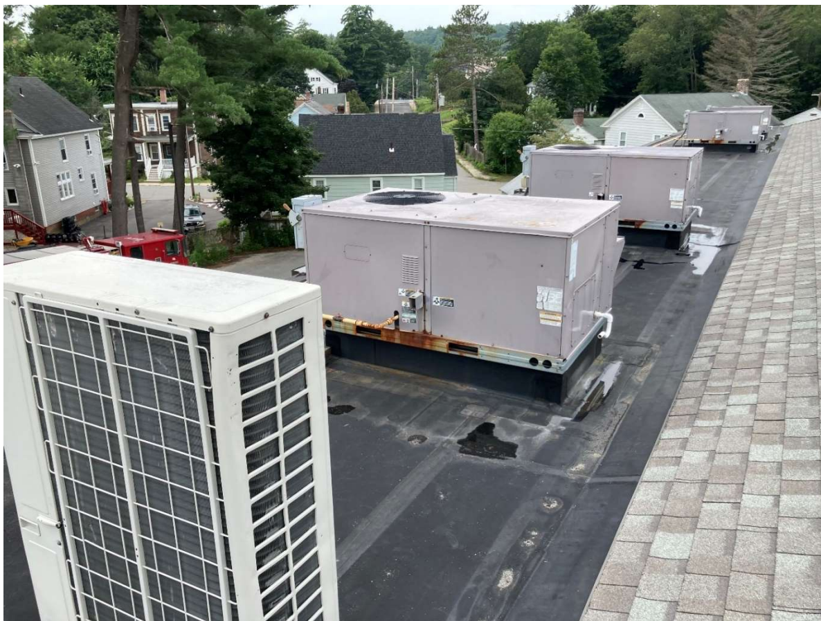
Picture 5: There are four (4) RTUs and one (1) ductless split unit located on the flat section of the roof.
