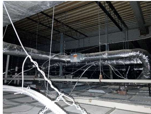
Pictures 6 & 7: Warren electric resistance duct reheat coils located above the drop ceiling.
