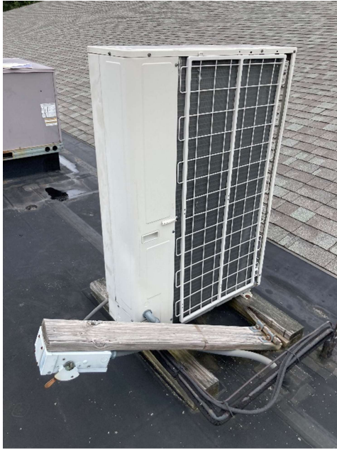
Pictures 8 & 9: The broken disconnect support at the Daikin ODU and the deteriorated pipe insulation.
