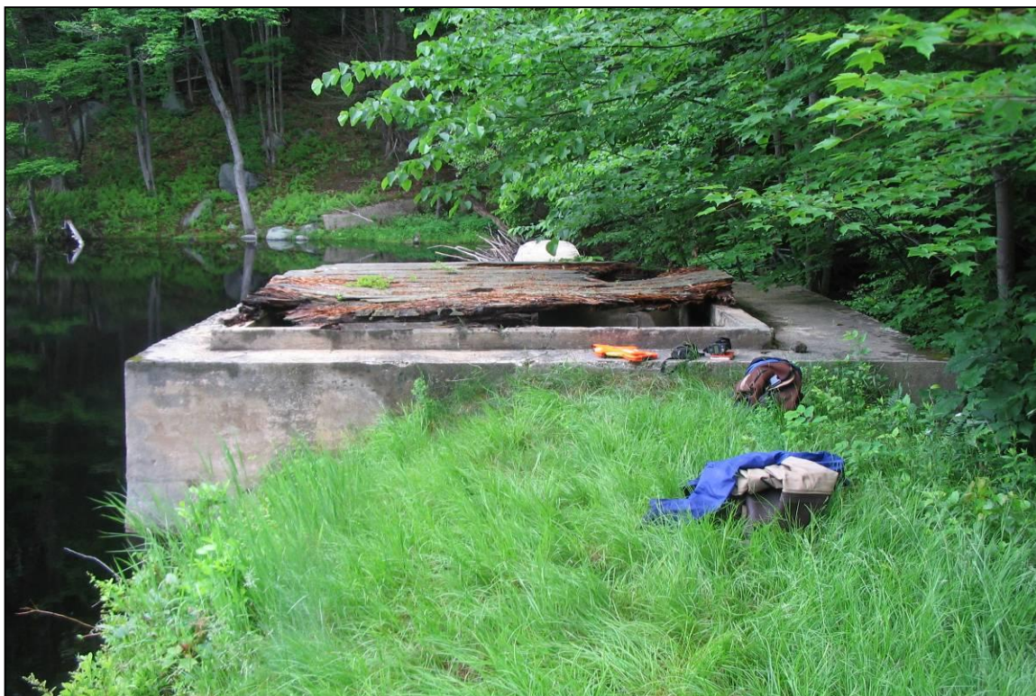
Photo 4: Intake chamber, note rotted lid
