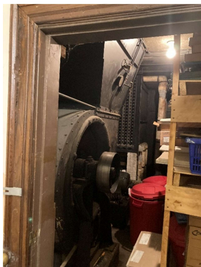
Picture 18: Disconnected original heating and ventilation unit for the Memorial Hall.
