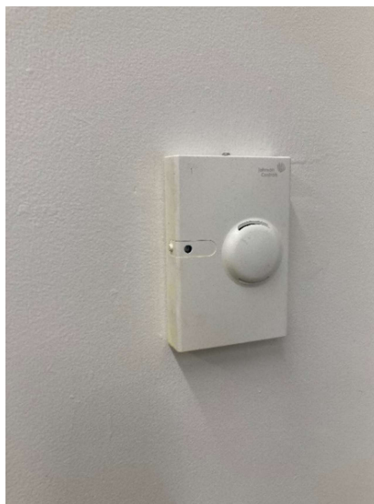
Picture 19: A wall mounted temperature sensor.
