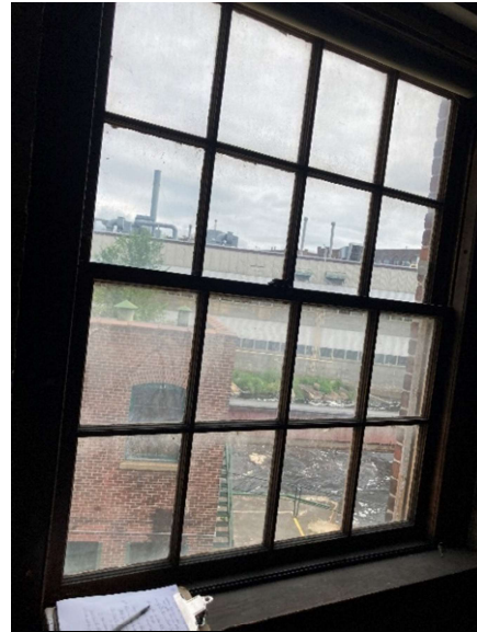
Picture 7: Typical wooden framed, single pane double hung window.
