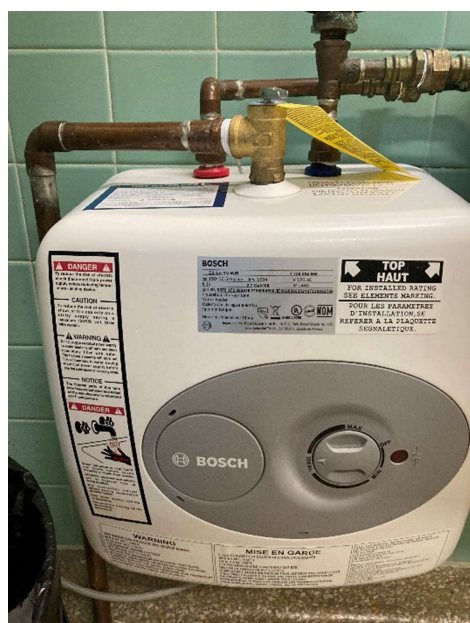
Picture 16: Small water heater in a restroom.
