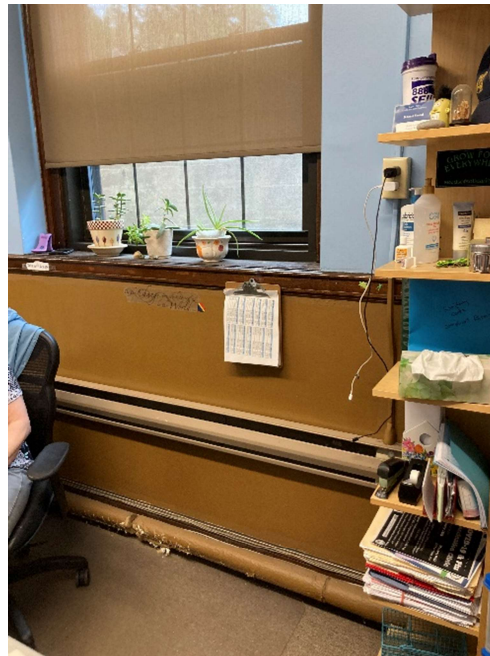
Picture 21: Electric baseboard heat
