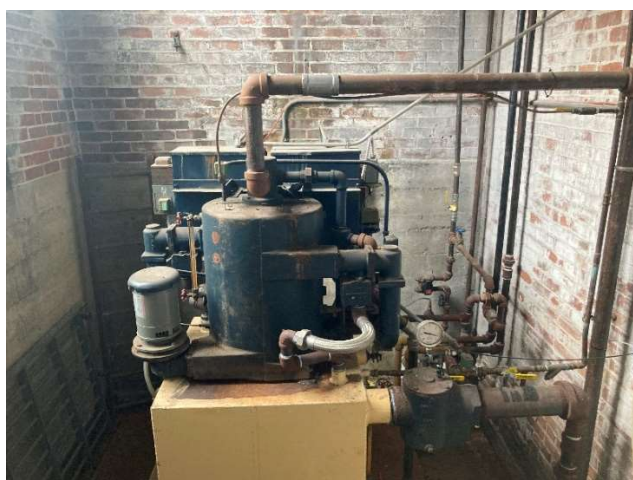
Pictures 9 and 10: The oil-fired steam boiler and the condensate return tank and pumps.
