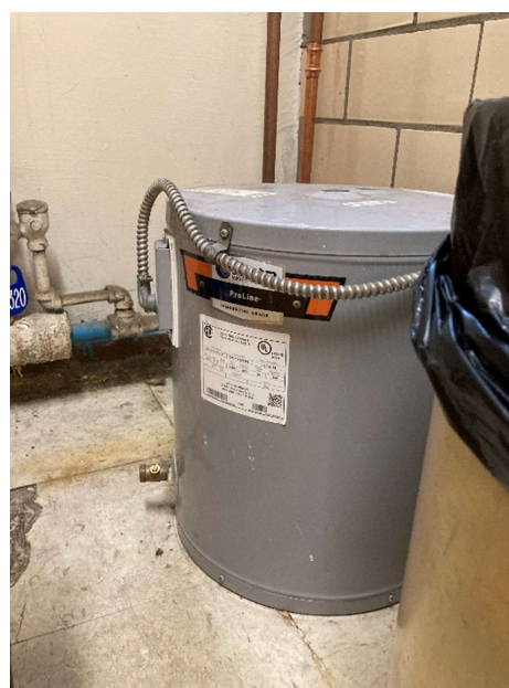
Picture 17: Electric water heater in Janitor's Room.
