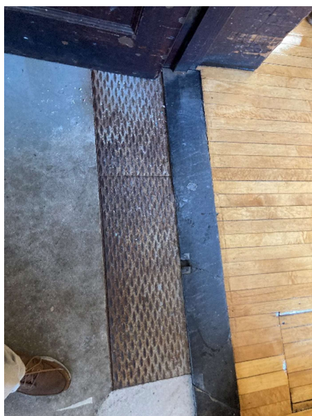
Picture 14: Steel covers over the trench piping.
