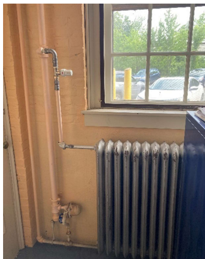
Picture 11: Kitchen radiator and piping. Pictures 12 & 13: Radiator with insulated piping and recessed radiator.
