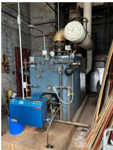
Pictures 9 and 10: The oil-fired steam boiler and the condensate return tank and pumps.
