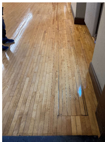
Picture 15: Removable floor sections over trench.
