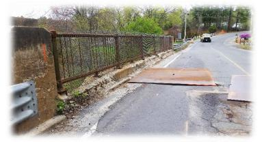
The "secret bridge" under Crescent Street is separate from the main bridge replaced last year with state funding. This sluiceway is north of the main bridge and carries a portion of the Millers River directly under the Starrett complex.
